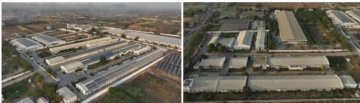
Wiring Harness and Electronics plants at Farola, Aurangabad
